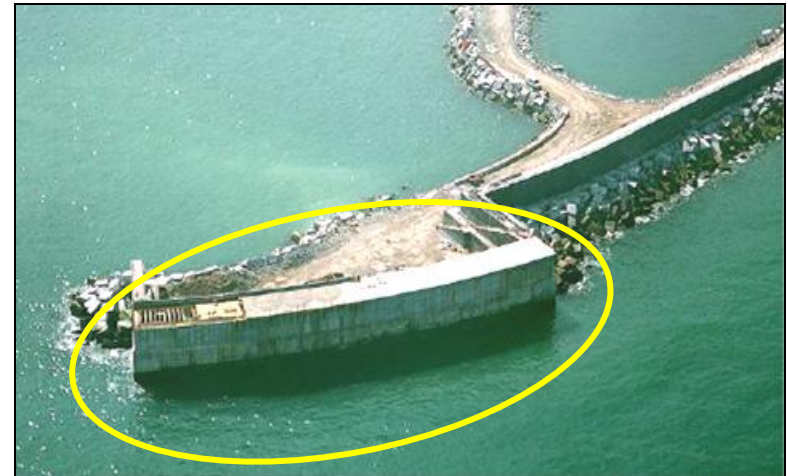
16 OWCs integrated into breakwater, Mutriku (Spain), 2008.
