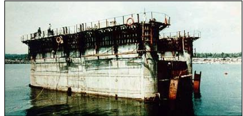
Construction in yard; towed and sunk into place (India), 1990
