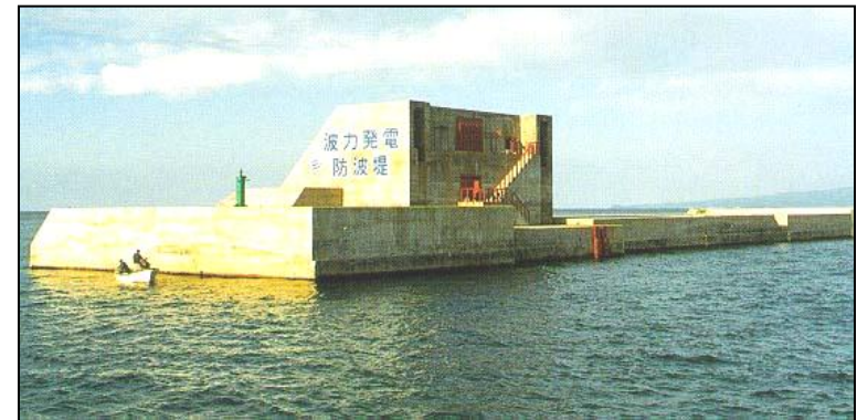
OWC integrated into a breakwater, Sakata, Japan, 1990.
